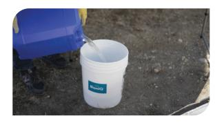
5. Mix thoroughly with a paint mixer or a squirrel cage attachment until all the powder has dissolved. Additional mixing time is required if using manual instruments.
